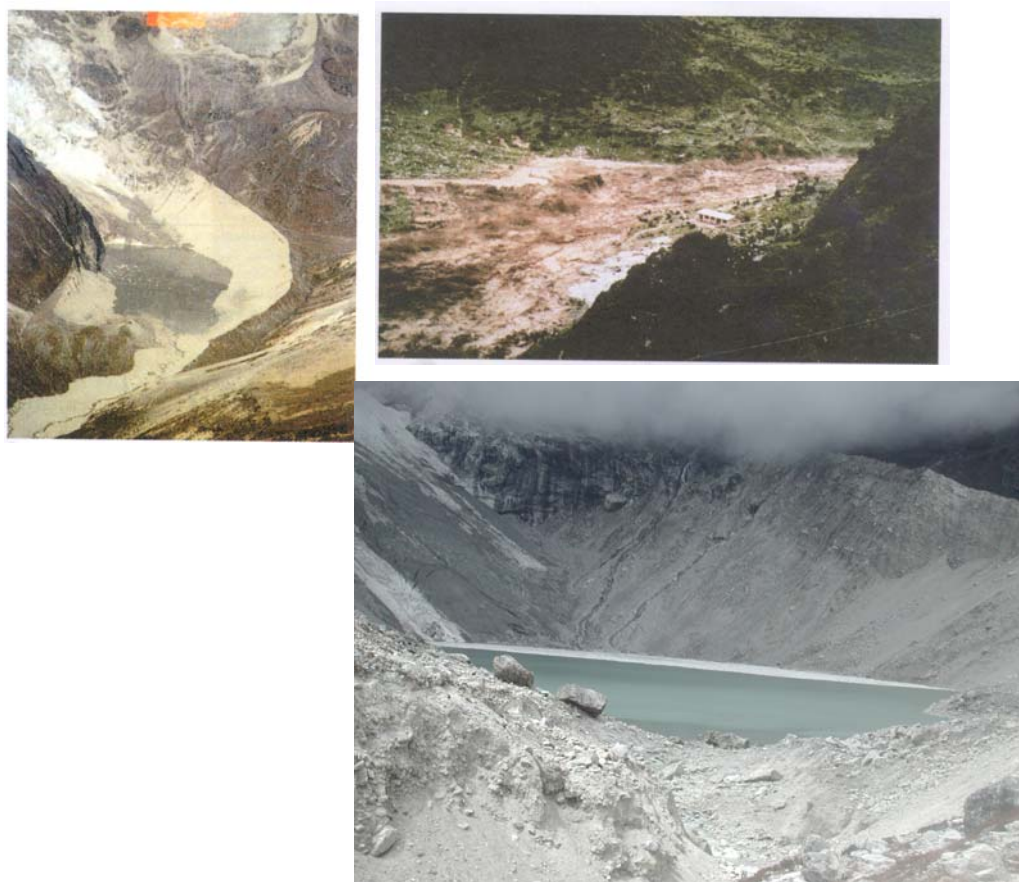
Figure 16: The Dig Tsho GLOF: The site of Namche Hydropower Project destroyed by the GLOF on 4 August 1985 (left) ( Source: WECS). The lake in 2004 (bottom) (Source: WWF Nepal Program)
